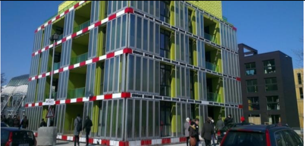
The BIQ House: the first algae-powered building, IMAGE © COLT INTERNATIONAL
